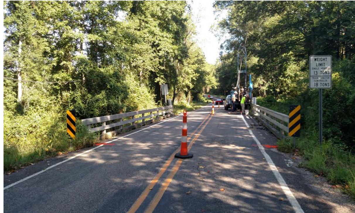
View of Existing Bridge No. 013 Looking Upstation
