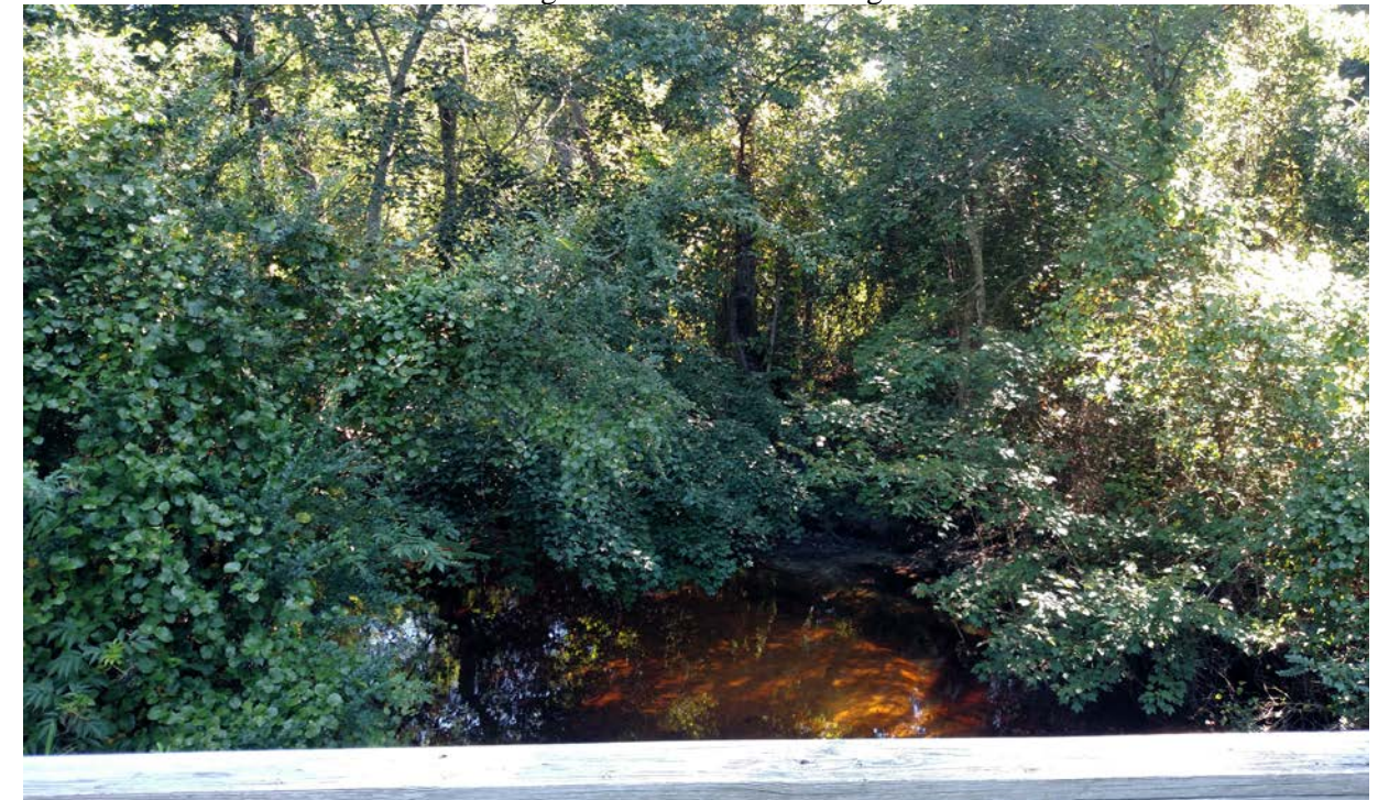
View Looking Downstream from Bridge No. 013
