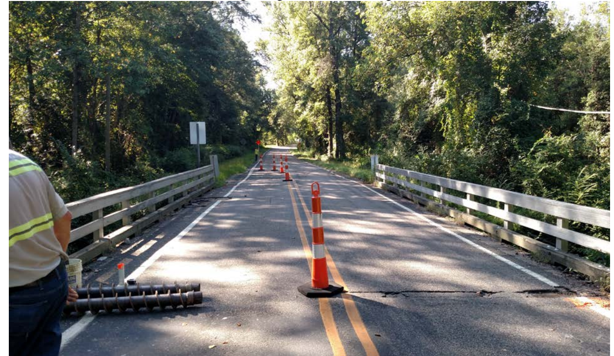
View of Existing Bridge No. 013 Looking Downstation
