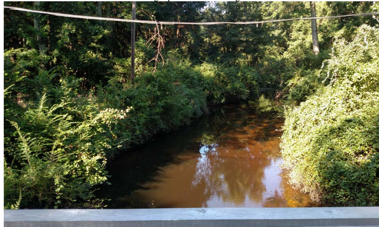
View Looking Upstream from Bridge No. 013
